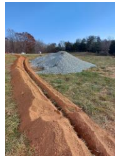
Above: Pipeline trench for an SL-6 fencing & water system
